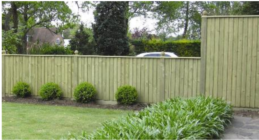
Treated pine lapped - Typical internal side fencing between units if required and to western boundary if required.
